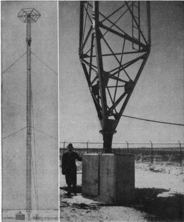
FIG. 2.55. A top-loaded sectionalized guyed vertical radiator and its base detail. Radio Station WMAQ, Chicago, Illinois. (Photograph courtesy of National Broadcasting Company.)
