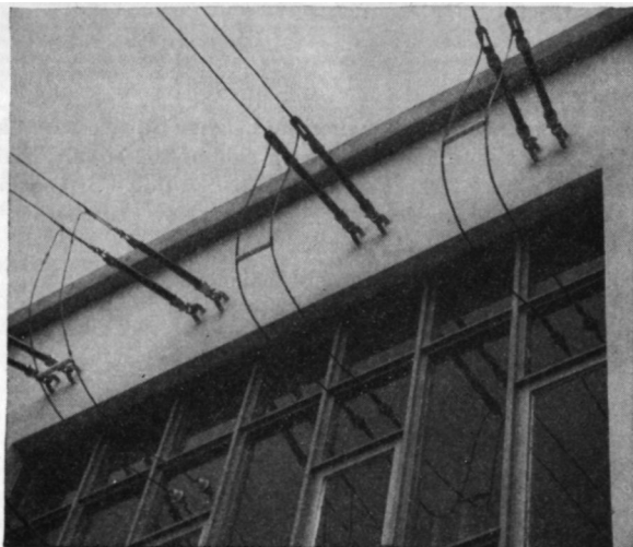
FIG. 4.96. Building entrance detail for several two-wire balanced feeders. (Photograph courtesy of Canadian Broadcasting Corporation.)
