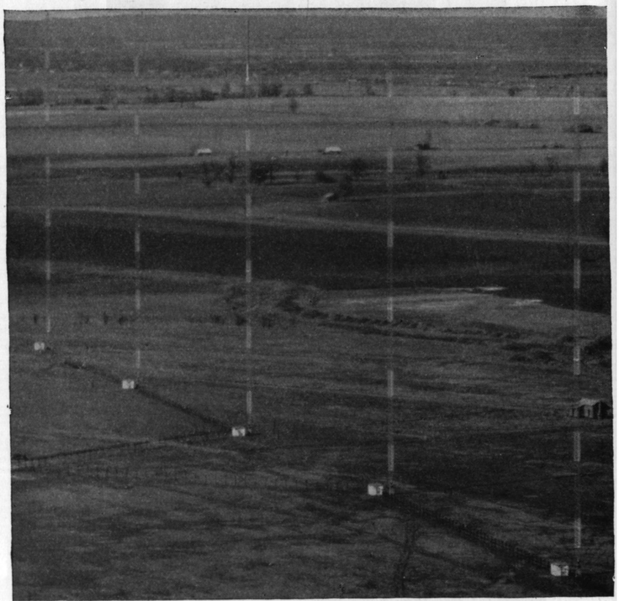
FIG. 2.66. View of Station KTBS six-element directive array. Note pylon antenna for frequency modulation on top of third radiator from the left. ( Photograph courtesy of W. M. Witty, Dallas, Texas. )
