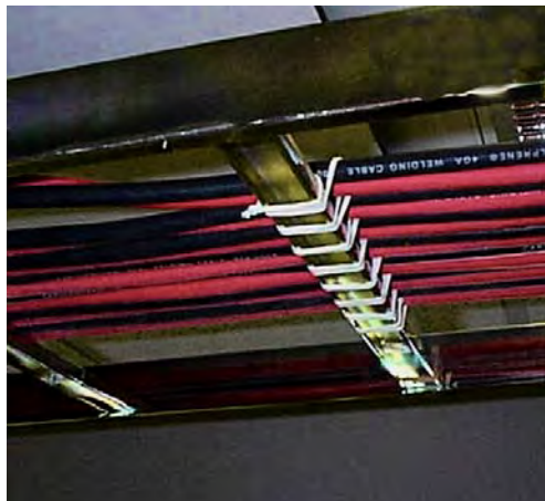
FIGURE 9-17 TELEPHONE COMPANY LACING METHODS
