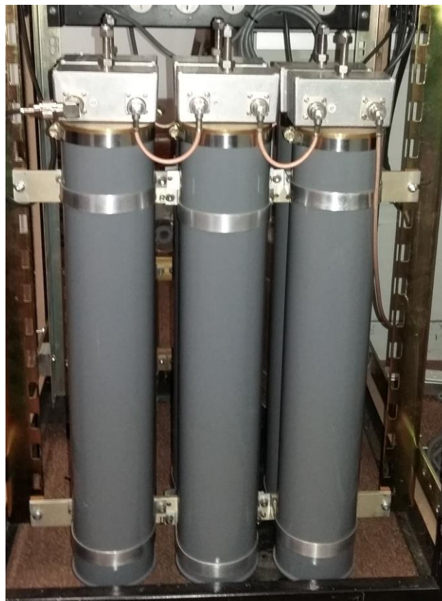
The completed duplexer in its final installation
