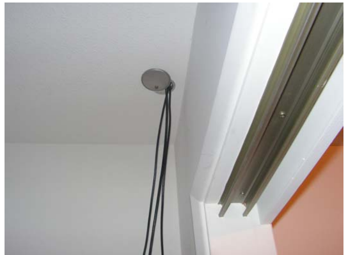
Figure 5 — To get the coax out of the attic crawl space and into the bedroom where the station is located, a 2 inch hole was drilled in the bedroom closet ceiling. Another attic vent, modified by adding a moveable cover, was used to finish the job.
