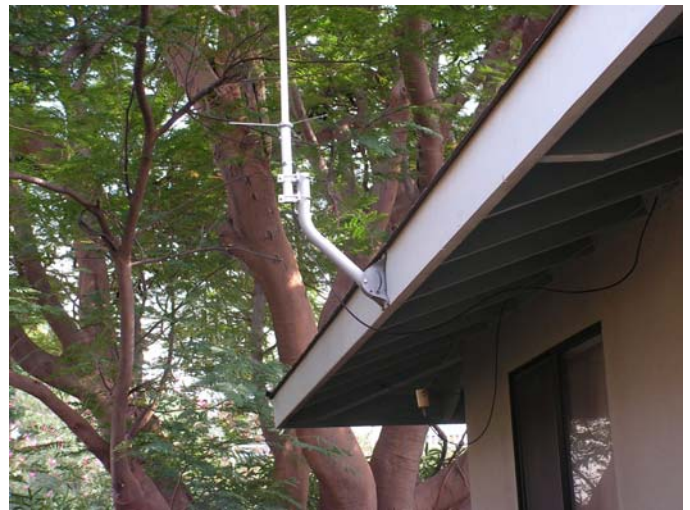
Figure 1 — The J-pipe mount commonly used for supporting DBS dish antennas makes an ideal mount for small amateur radio antennas. The one shown here mounts a dual band antenna to the fascia board of a house.
