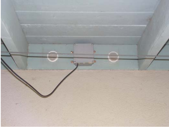
Figure 2 — The center attic vent was removed and a box was installed over the existing hole. This permits the coax to enter the attic crawl space while keeping the bugs out.
