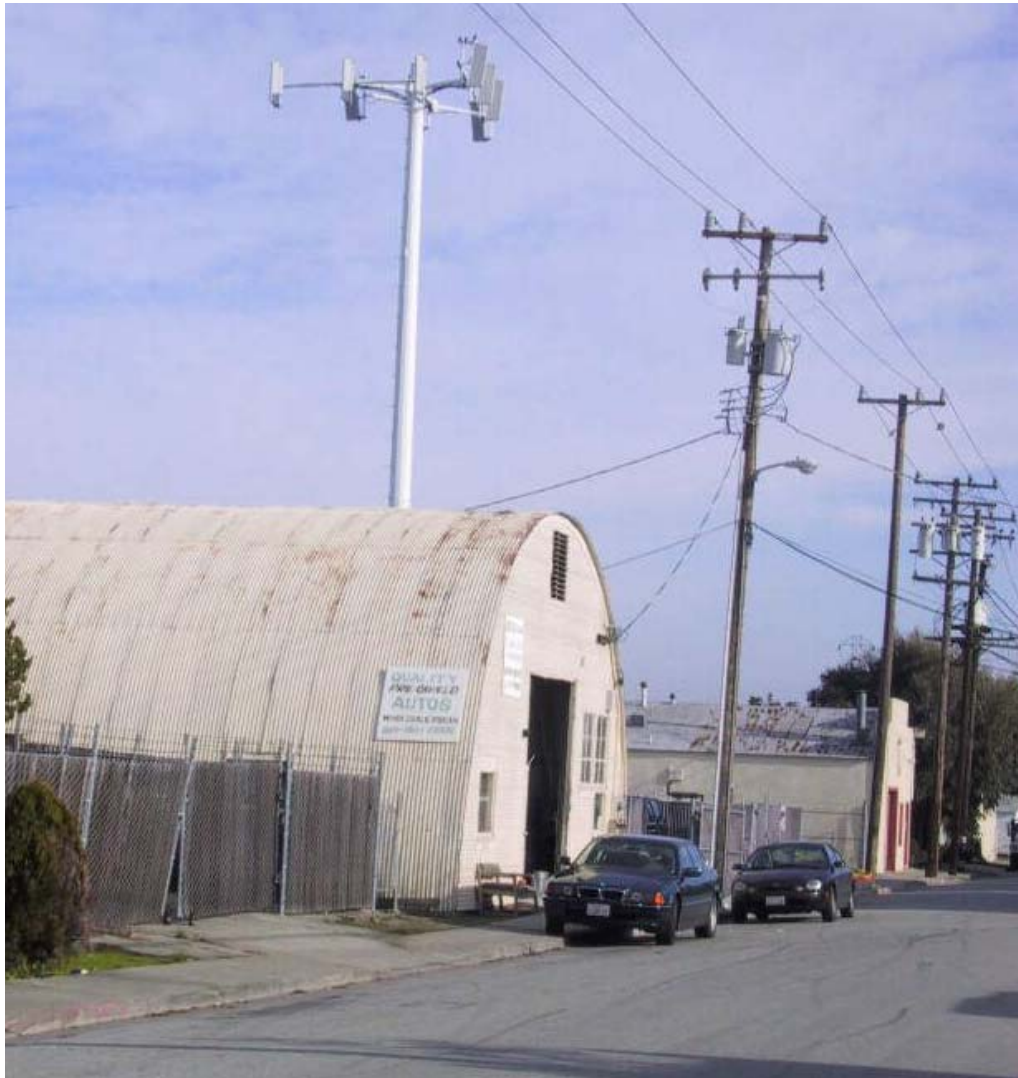
Figure 37 - 40 Ft Tower with Down Tilted Directional Antennas
