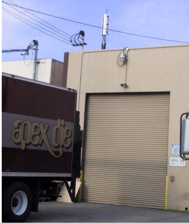
Figure 38 -Directional Antennas On One Story Building
