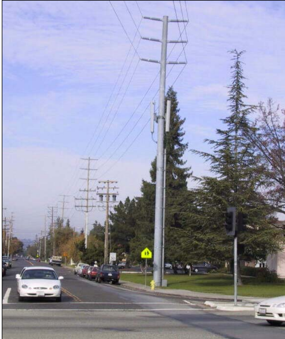
Figure 40 - Directional Antenna Site on Power Pole
