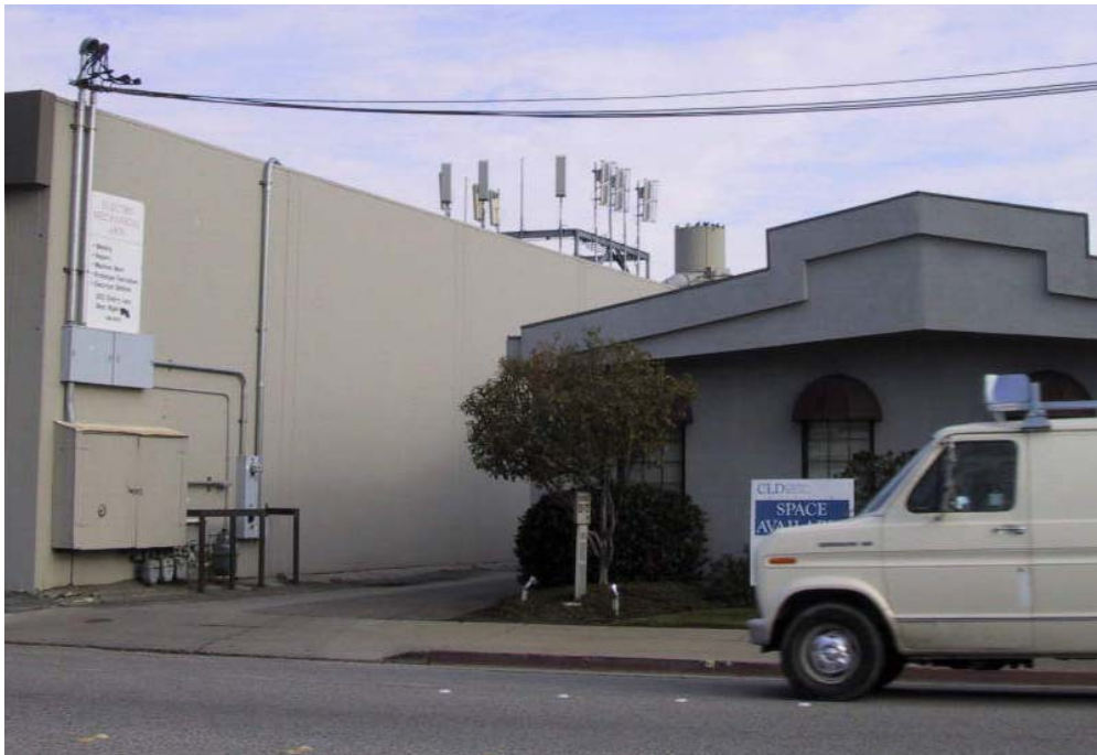
Figure 39 - Adjacent Building. Down Tilt Antennas
