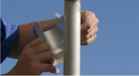
Step 7: Use the half-round file to de-burr the inside of the sleeve. Extra filing will be necessary if the end of the sleeve has been distorted by the pressure of the tubing cutter wheel. File as necessary until you are able to insert the plastic spacer at least part way into the sleeve:
