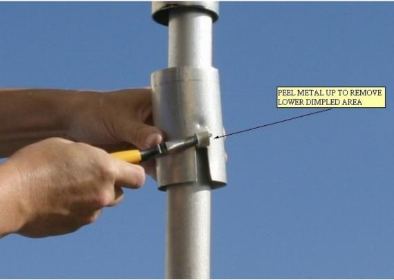
Remove material as necessary to allow removal of the plastic spacer without stressing it and causing cracks. Slide the spacer down the mounting pipe and out of the way. Cut the rest of the way through the excess sleeve piece and remove it from the mounting pipe:
