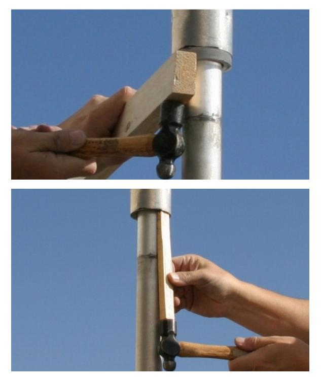
Step 10: Make two dimples under the plastic spacer, one on each side of the sleeve, to hold the spacer in place. Insert the tool until it touches the spacer, then back off 1/8 inch or so and make the dimple. This keeps the tool from scratching the spacer.
